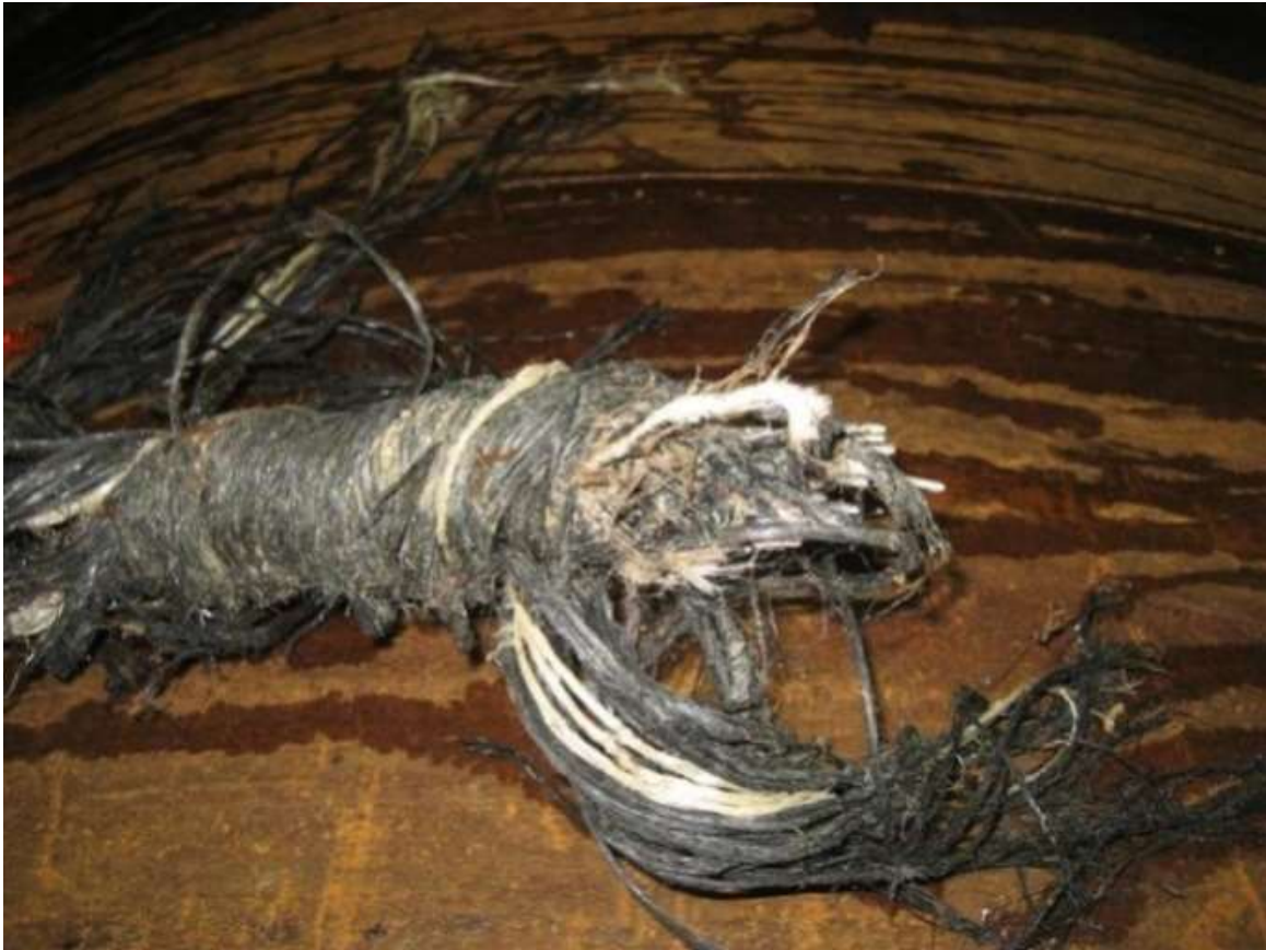
A frayed and severed cable, cause unknown [5]
